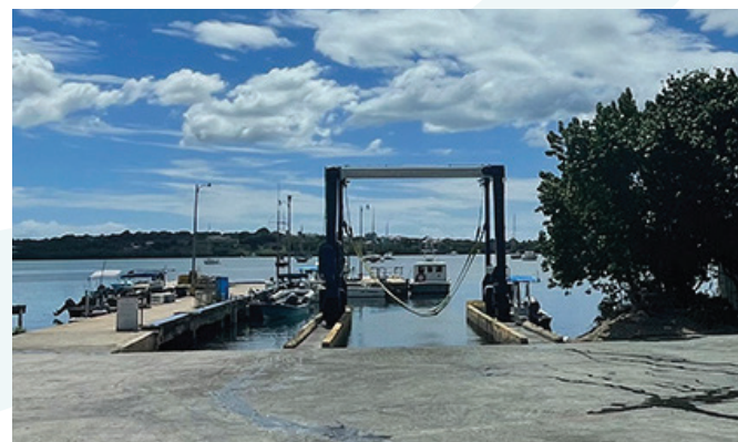
Picture 55. Ramp Area
